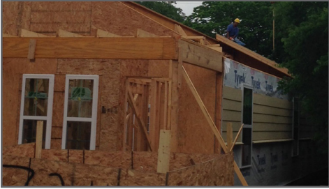
Tarrant County Housing Partnership teamed up with the City to build one of the city's first homes using a Structural Insulated Panel system, which creates tight, well-insulated, housing structures that resist fire, wind, insects, and decay. The panels for this home were purchased from Korwall Industries, Inc., located in Arlington. Funding for this project was made possible by a City of Arlington HOME grant.
